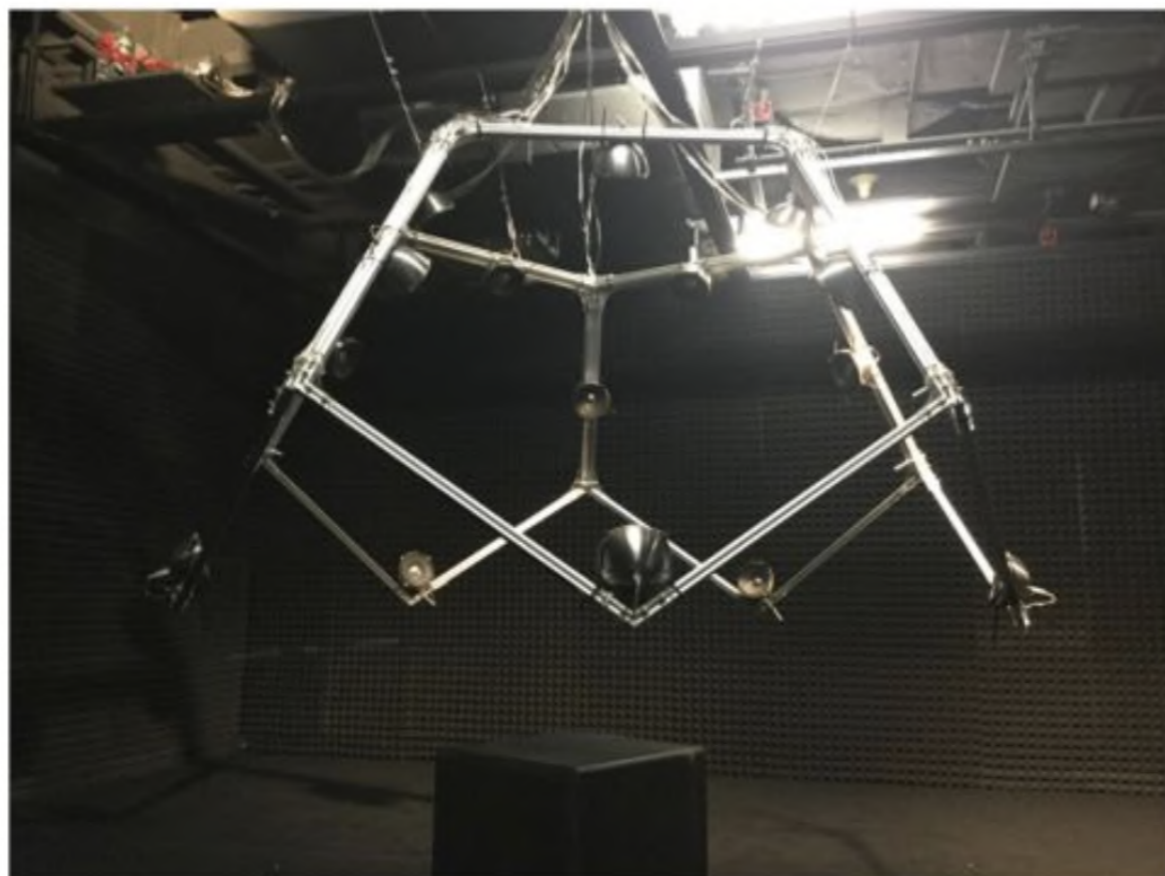
LOKI structure suspended above subwoofer. Note the equipment platform in the grid, above to the left.
